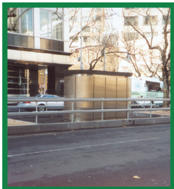
Rear view - central city location
