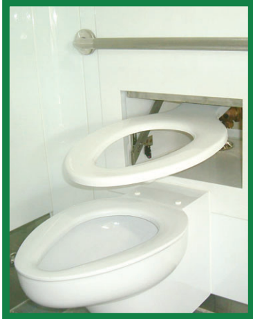
Clean seat being lowered into position
